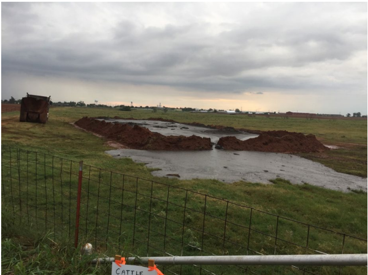
Figure 5 Temporary pit overflowing
