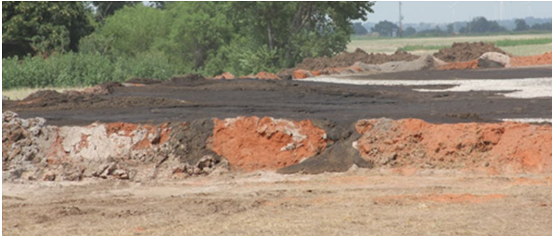
Figure 6 Temporary pit breach
